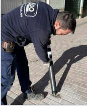
**4.** Let the resin dry (10 *minutes*) and then you can screw the bollard.
