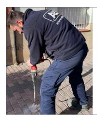
Make a hole in the ground in order to place the anchorage.
