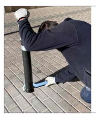
**5.** Screw the bollard with the help of the key (not included).
