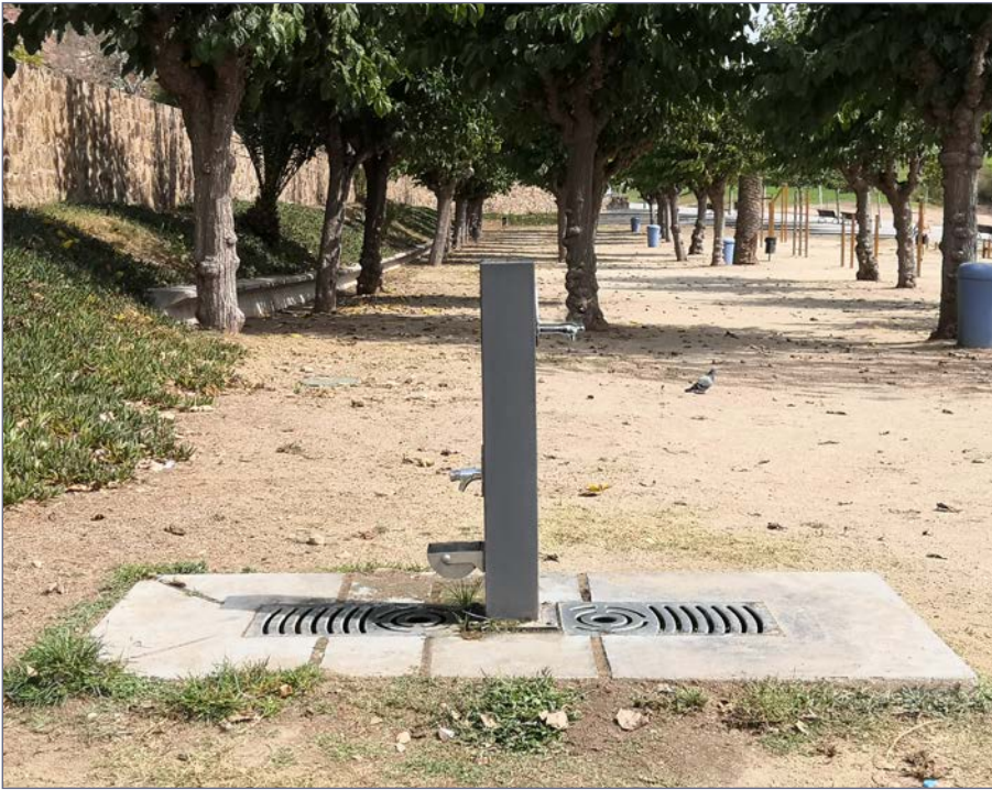
Detail lower tap and later emptying of the trough for animals.
