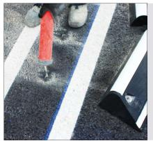
**3.** Remove the separator and clean the holes of waste.
