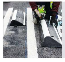
Place the separator with the threaded rods and nuts. **Ref. MOMPETOR**
