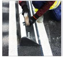
Wait until the resin is dry and adjust the separator with the nut.
