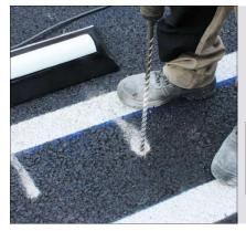
**2.** Drill with a Ø14 bit to the indicated depth in each one of the fixing holes.
