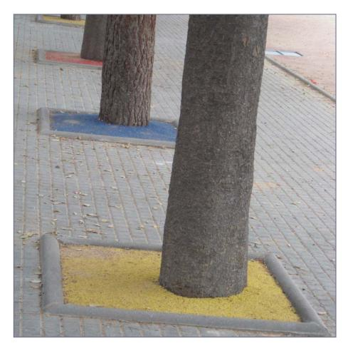
Recycled rubber tree pit in different colors to choose from. It is placed in different layers of different granulometry adhered with resin.
